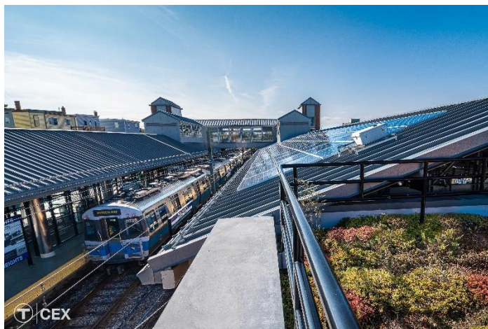
Photo 6: Solar panels at Orient Heights station
