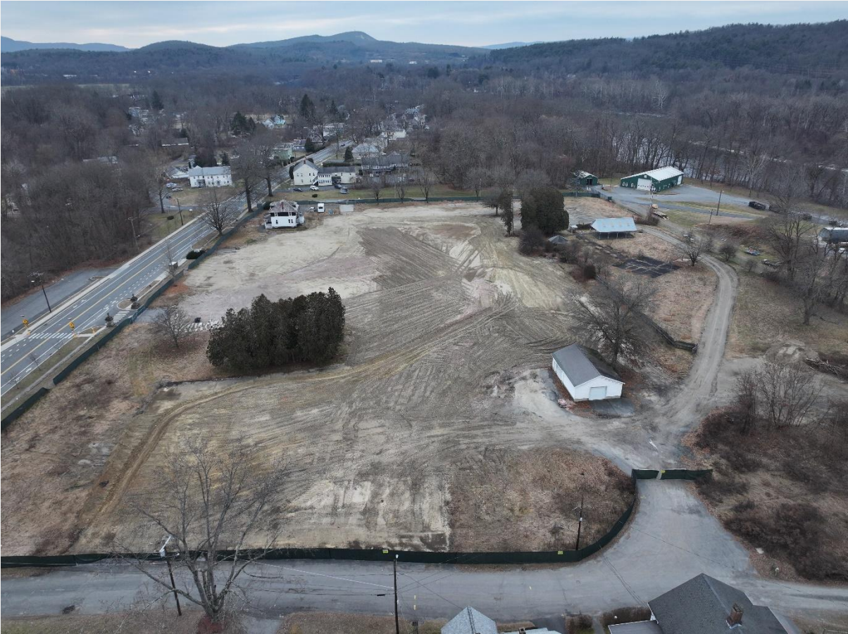
Former Farren Care Center site, post-demo, now owned by Town
