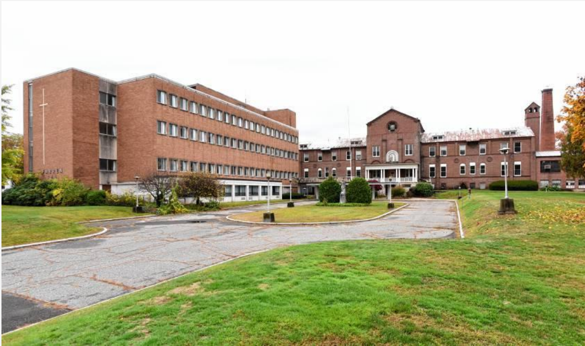
Former Farren Care Center buildings, before demo
