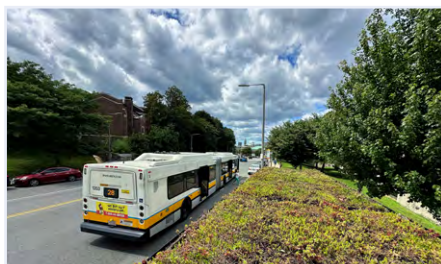
The city of Boston has installed green, vegetation-covered roofs on 30 bus shelters along a popular route to provide cooling and help manage stormwater. (Photo courtesy city of Boston/Trevor Smith at Weston Nurseries)
