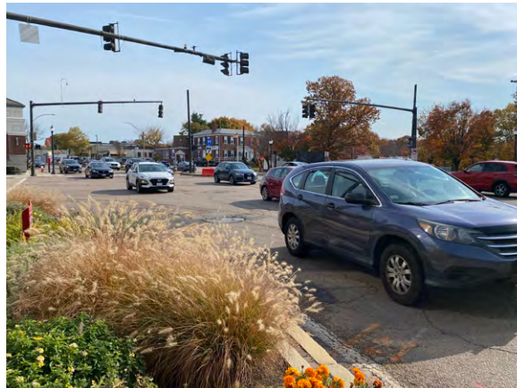
Funds from three federal traffic programs will inject $12.4 million into road safety efforts across Massachusetts.
